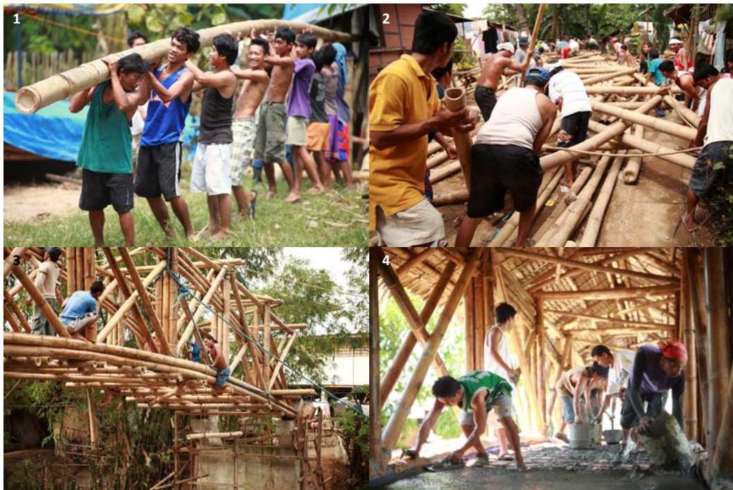
(1) Community members performing “Bayanihan”; (2) Assembling the structural component of the bridge offsite; (3) Assembling of the bamboo bridge; (4) People pouring concrete slab
