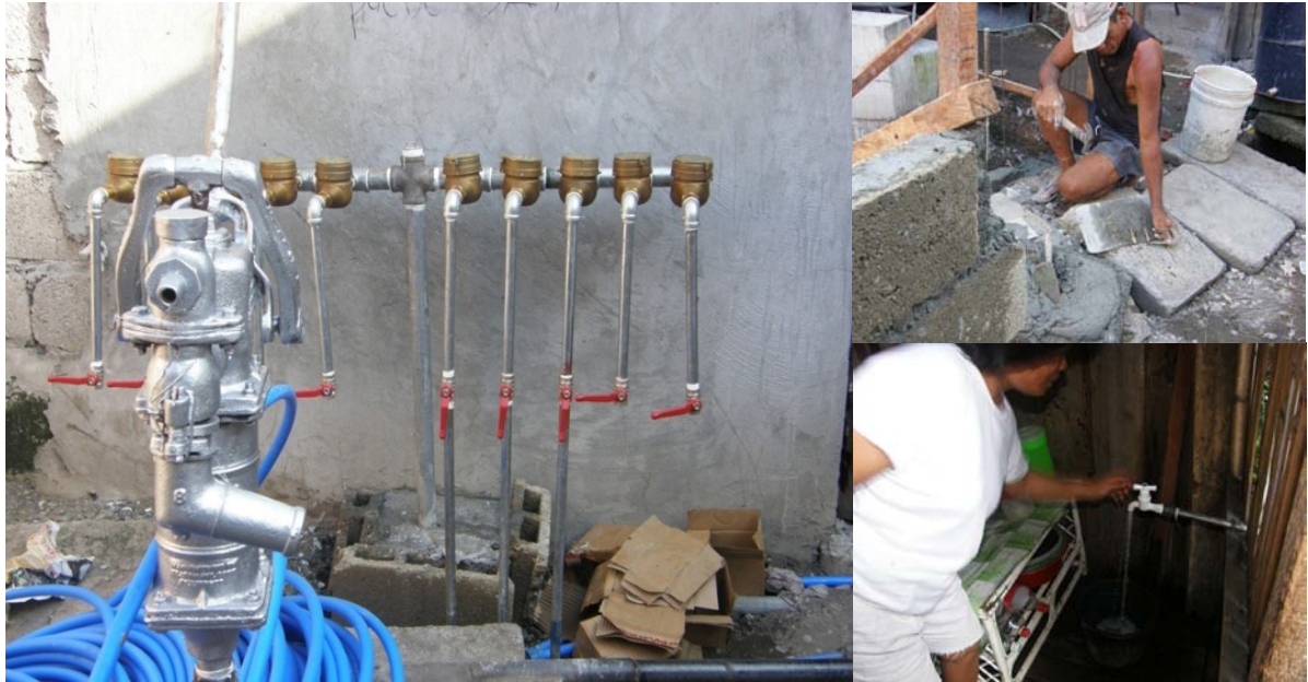
(1) Clustered water meters; (2) Construction of water system; (3) Water connection in house (Image Source: ASHAI)
