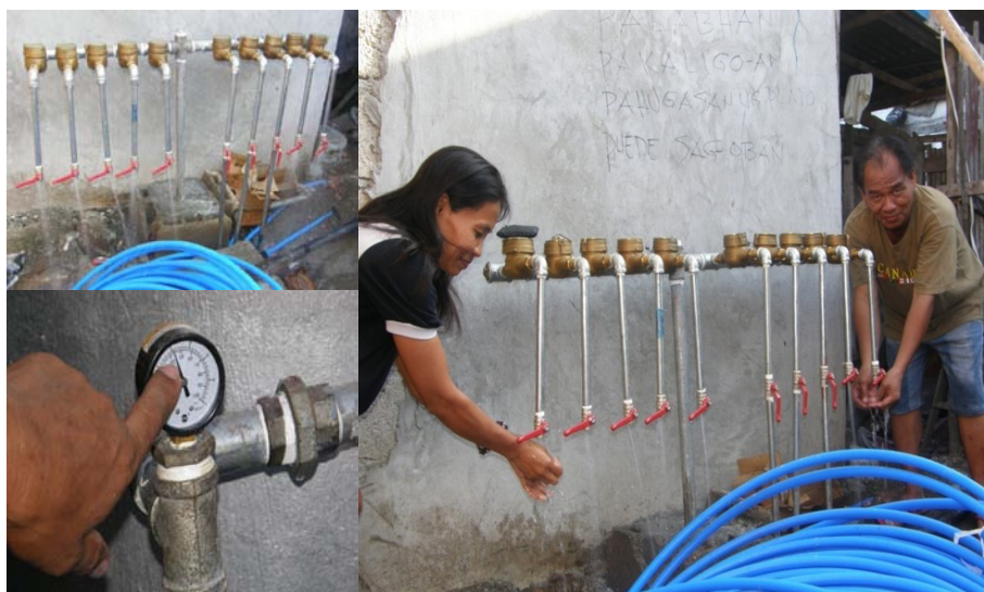
Clustered meters connected to the water pump
