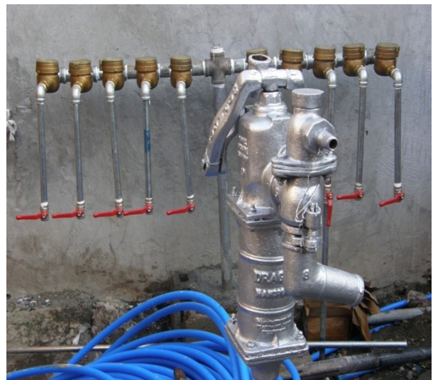
ASHAI water supply system connecting to the main water source going to every community household
